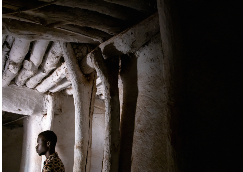
Iwan Baan (*1975) Grand Mosque, Bobo-Dioulasso, Burkina Faso, The ancient natural wooden construction typical of Sudan-Sahelian architecture, of which Bobo-Dioulasso's Grand Mosque is one of the few remaining examples, 2021 Photography © Iwan Baan
